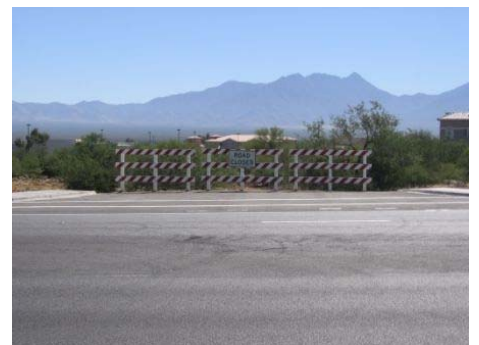
Pictured above is the site of the future Alpha Avenue/Duval Mine Road intersection, west of the I-19/Duval Mine Road interchange and just east of the Safeway.
